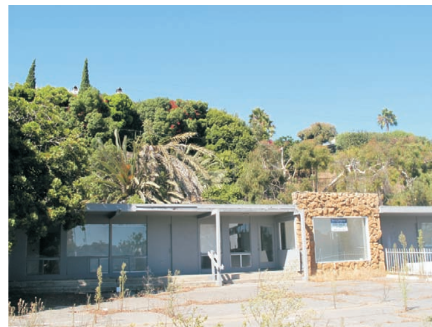
3 View of property looking north.
